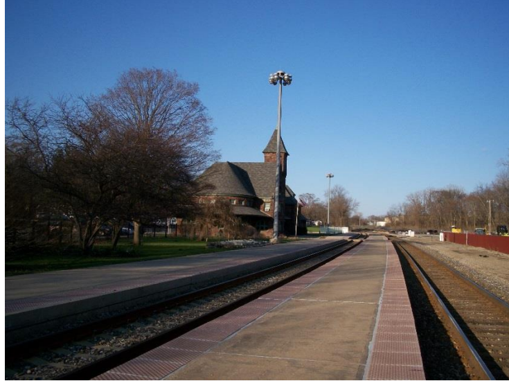
View of station building from center platform, looking east. Source: Author.
