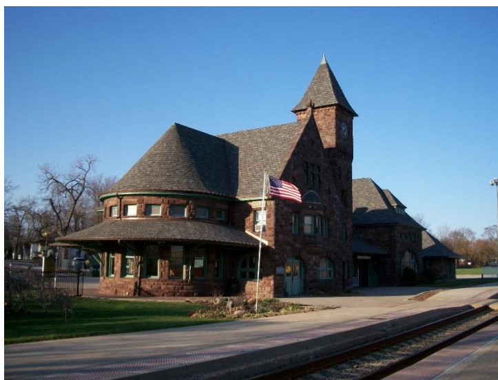
View of station building from platform. Source: Author.
