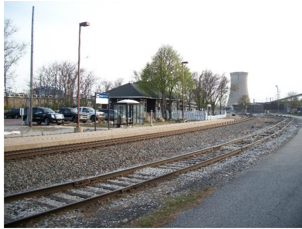
View of platform from across tracks, looking west. Source: Author.
