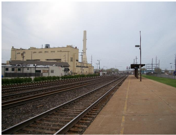
Hammond station platform, looking west. Source: Author.
